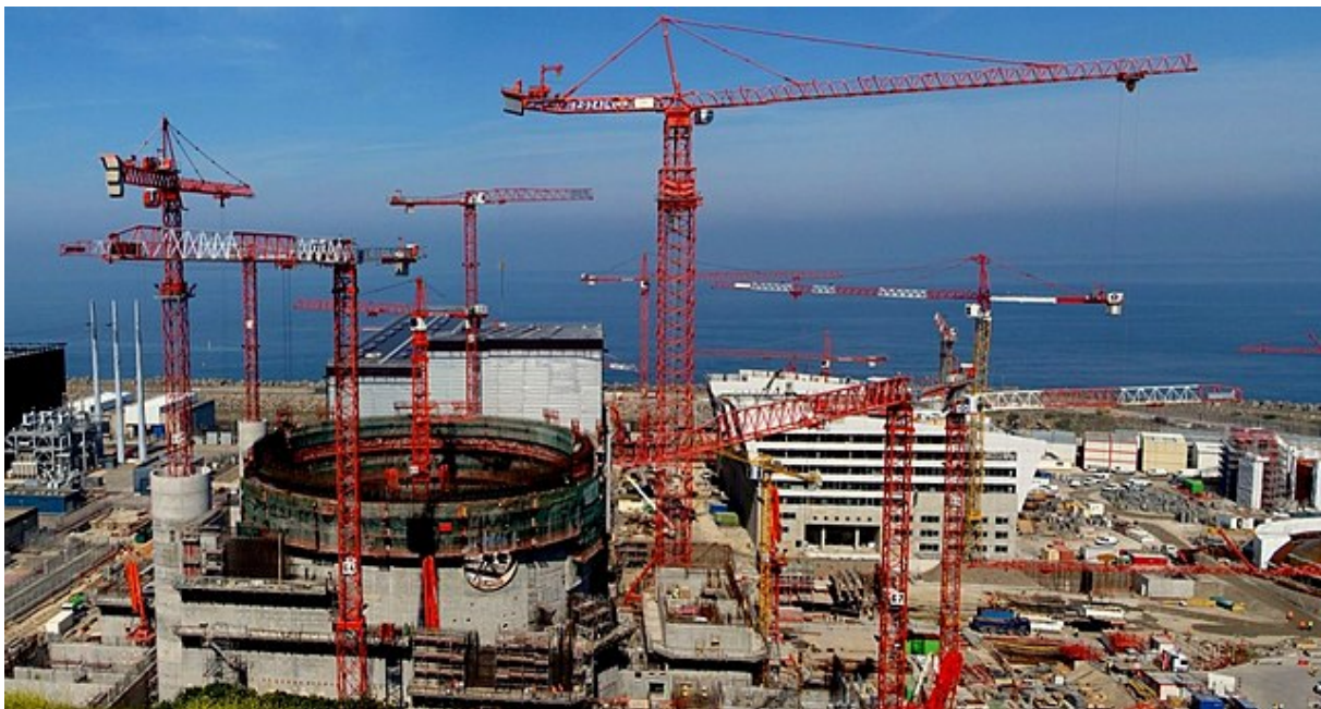
Figure 3.3.7-1. Unit 3 of Flamanville NPP under construction (France, 2010)
