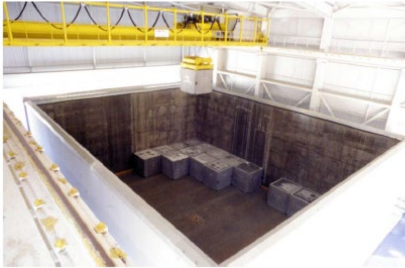
Figure 5.1-5. El Cabril near surface disposal facility, Spain.
