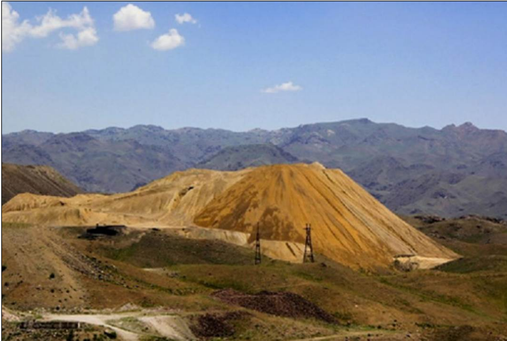
Figure 3.3.1-9. – Tailings at the Taboshar site (abandoned uranium mine in Tajikistan)
