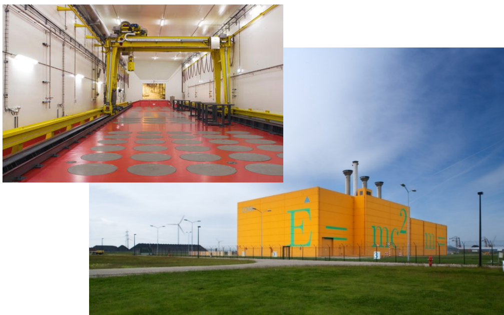
Figure 4.2-2. HABOG centralized HLW dry storage facility in the Netherlands.
